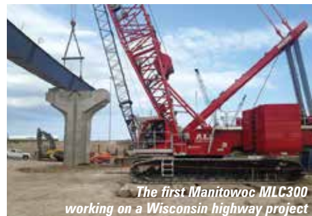
The crane was rigged with 48 metres of main boom and 172 tonnes of counterweight
