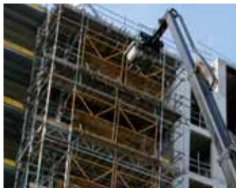
One of the Manitou MRT 2540 telehandlers placing materials on the upper floor.
