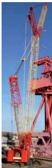
The Kobelco SL6000 working in the Weldex fleet
