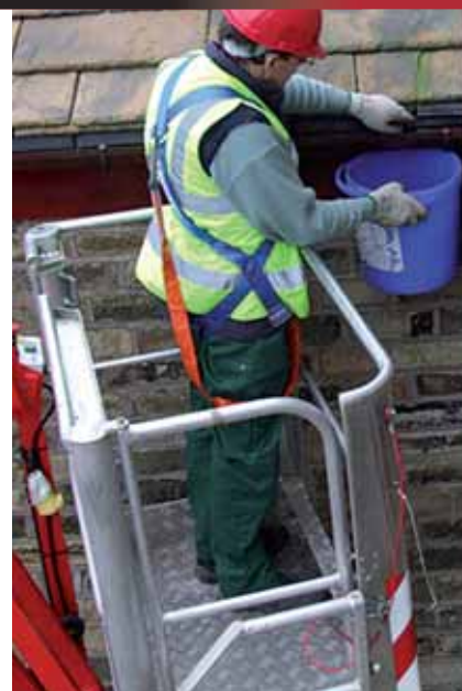
The truck mounted platform is kept very busy.
