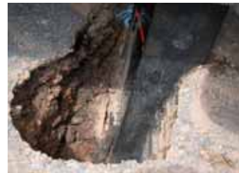
The ground looked OK on the surface.
