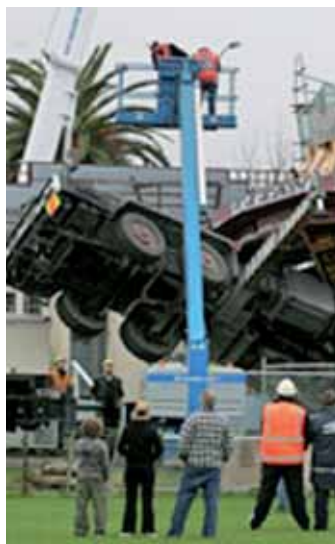
July 2007: A 50 tonne Kato NK500 truck crane, owned by Titan crane hire of New Zealand, had just started lifting steel roof trusses at a site in Taurenaga, when the ground gave way. It turned out was set up over an old septic tank which collapsed. The crane missed traffic on a main road but the boom caused extensive damage to the three-storey building and scaffolding. The boom had to be cut up to remove the crane.
