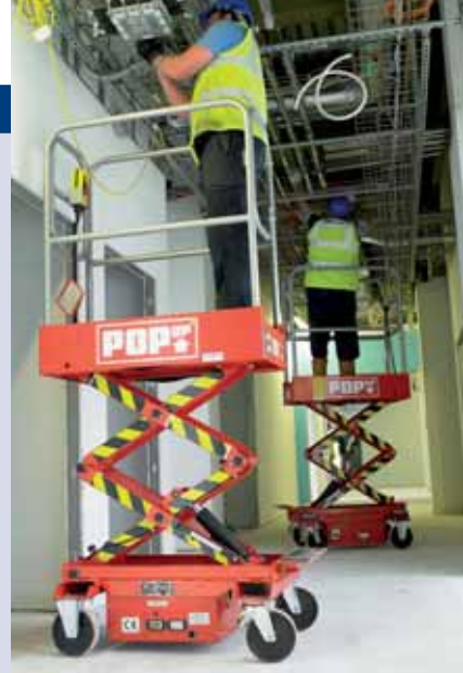
More than 75 Pop-Ups are working on the Birmingham New Hospital.
