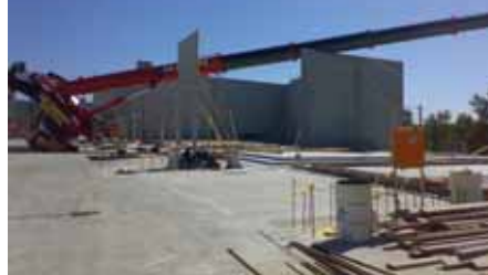
The crane tipped and the boom came to rest on a panel
