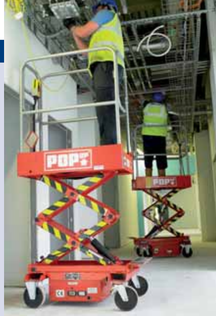
More than 75 Pop-Ups are working on the Birmingham New Hospital.
