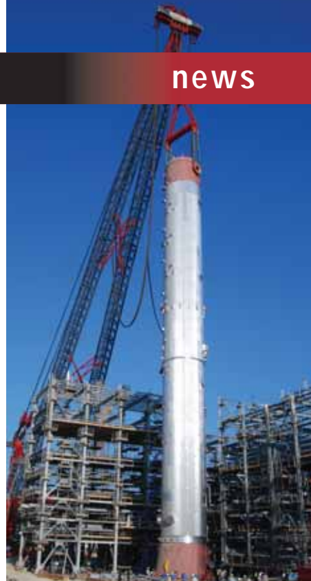
The ALE SK90 completes its first commercial lift - 755 tonnes at 84 metres.
