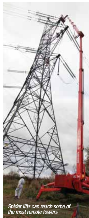
Linesmen in Denmark using a crane with platform and loader crane for transmission tower maintenance
