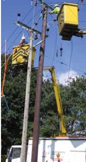
The preferred method of working on overhead power lines
