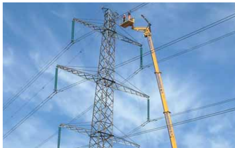
Linesmen in Denmark using a crane with platform and loader crane for transmission tower maintenance
