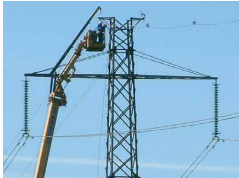
An alternative is to use a lift to place the trolleys which is proving to be faster and safer.
