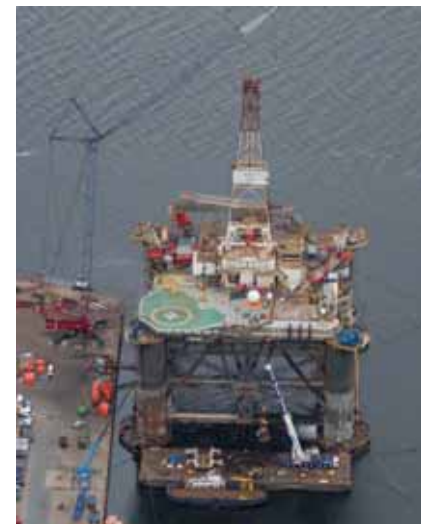
The 1,200 Gottwald AK912 was brought in principally to handle the rig's mast.
