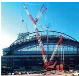
A CC12600 in action, currently the biggest Demag crawler crane.
