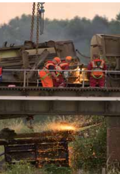
Workmen try to free the tangled trucks.
