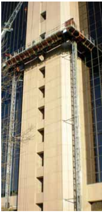
The Fraco mastclimber wrapped around the façade to provide full access
