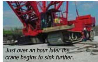
Aggregate platforms need to be carefully calculated and built or they can easily give way
