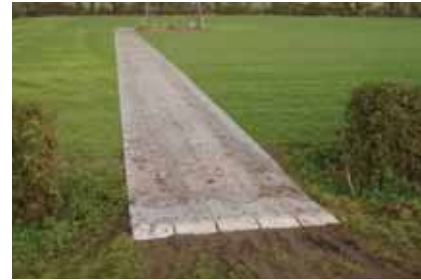
Aluminium road ways from companies such as TPA, Eve and Timbermat are well suited for wheeled cranes and lifts to gain access over soft ground.
