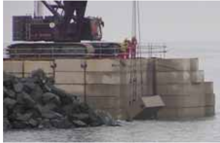
Our Heavy duty platform protection mats.
