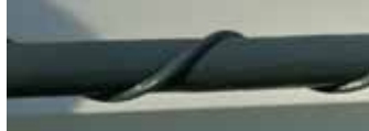
The carbon fibre pendant has a built in Helix to deflect wind.
