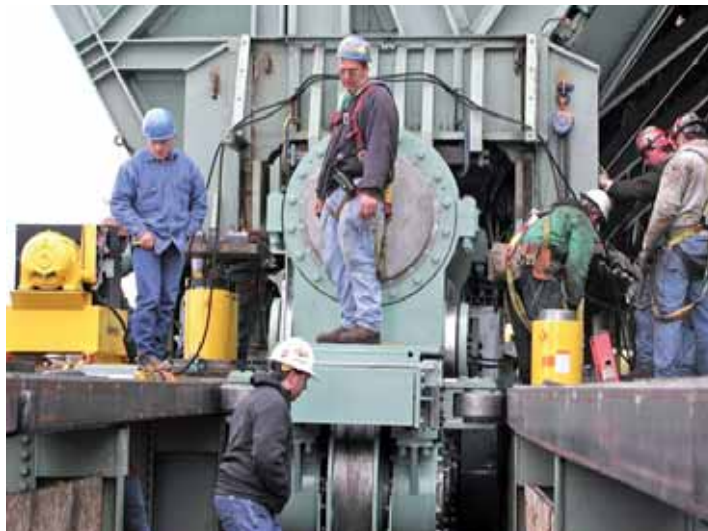
A new bogie in place. One wheel and two guide rollers are visible.
