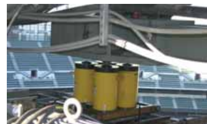
In this lift, the hydraulic jacks were arranged in a quad-cluster, fitted with spherical load caps and resting on a Teflon 'sandwich' to allow for lateral movement.
