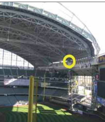
The roof is being lifted at the point circled in order to replace a bogie.
