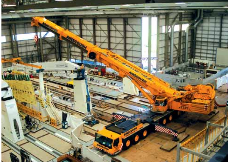
Ainscough's 500 tonne Liebherr working under cover.
