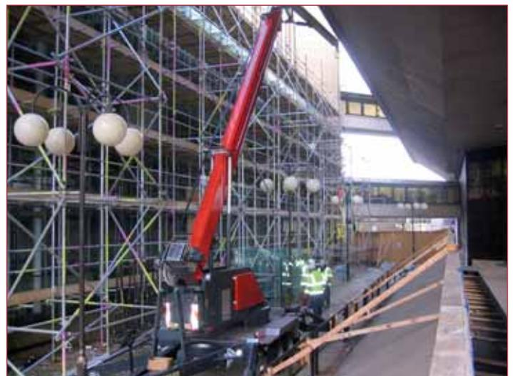
GGR was able to provide the Royal Bank of Scotland with a Skyworker crane after several other crane companies had to turn the job down. The Skyworker overcame restricted access problems and the need to reach over the top of the building to install the canopy glass.
