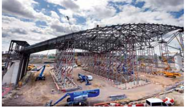
Up to 15 big booms - 125ft JLG 1250 and 135ft Genie Z135s from Hi-Reach are being used to erect the steelwork on the unusual wave shaped Aquatic Centre for the London Olympics.
