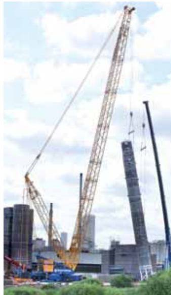
The Demag places the columns on top of the air separation facility
