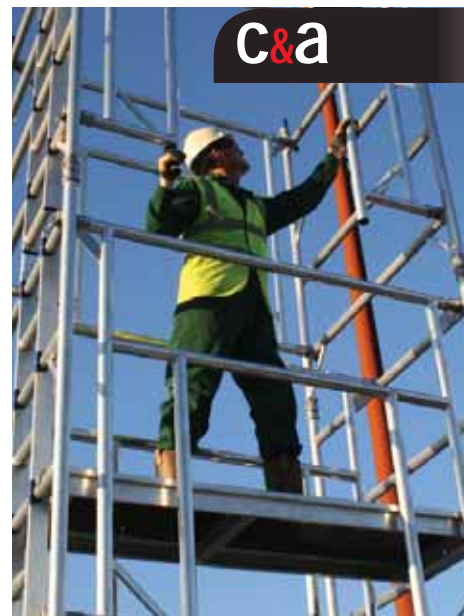
Advanced guardrails are fitted from below.
