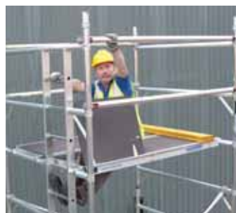
Installing the guardrails above through the trap door
