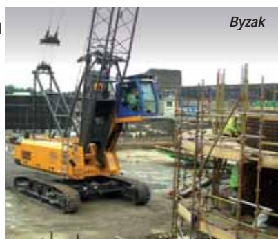
The Sennebogen 660 works on cantilevered falsework to carry out a wide variety of tasks
