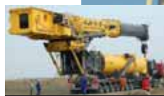
The Grove GTK1100 at work in outer Mongolia
