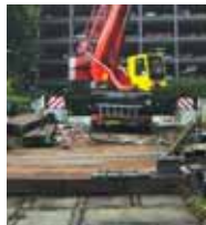
Heavy duty crane access mats
