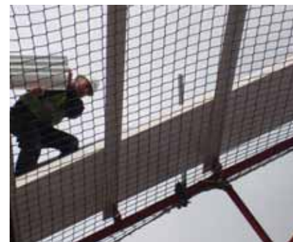
Men working above a well installed square mesh knotless net
