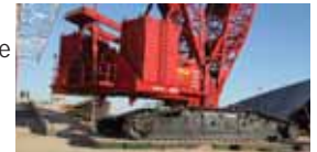
emtek mats providing a stable base allowing a 160t lift to be completed safely
