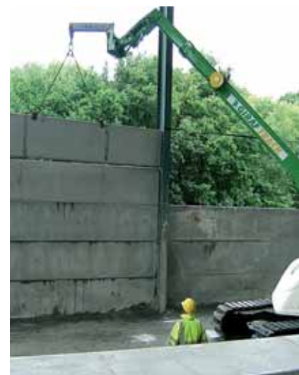
The Giraf Track can lift up to 3.8 tonnes.
