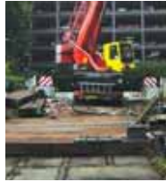
Heavy duty crane access mats
