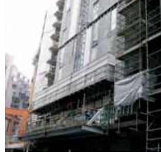
A single mast 40 metre high mastclimber runs from the first floor, leaving the ground floor unobstructed.
