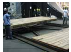
emtek mats manufactured to fit into a specifically designed steel frame
