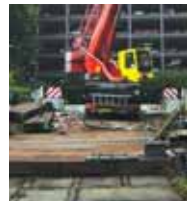
Heavy duty crane access mats
