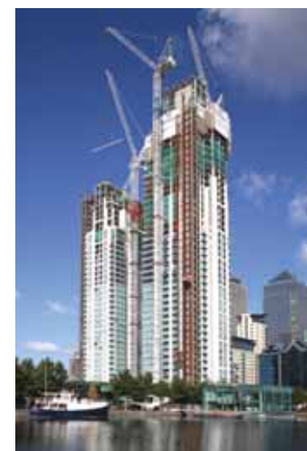
The Pan Peninsula development in Canary Wharf, London.
