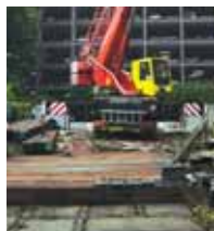
Heavy duty crane access mats
