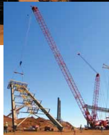
Monadelphous's new Manitowoc 18000 lifts a steel sub assembly.
