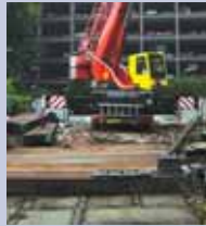
Heavy duty crane access mats
