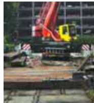
Heavy duty crane access mats
