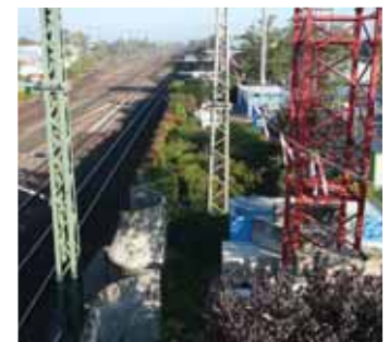
The MTT tower is set up close to the tracks.
