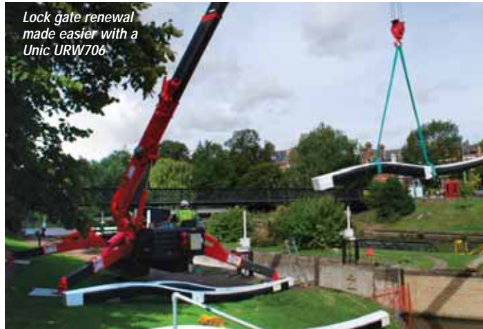
A mini crane can often find a way into lifting position
