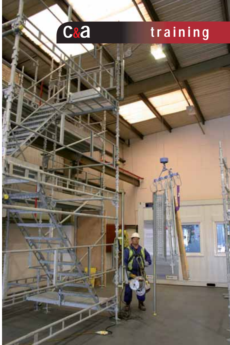
The electric winch allows several items to be lifted safely at the same time.
