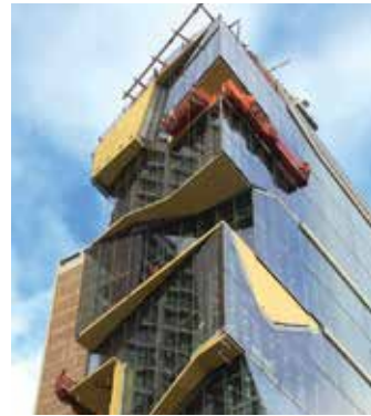
A monorail system and a material hoist worked in conjunction to safely manoeuvre the panels into position
