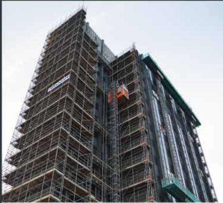
Double Stacked Mast Climbers Archway Tower
