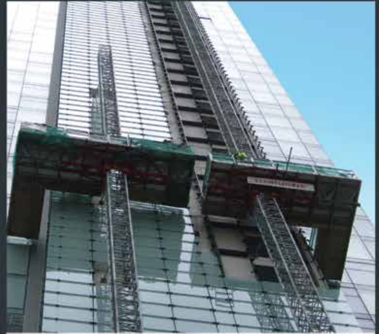
Heavy Duty Mast Climbers Tower West, Liverpool
