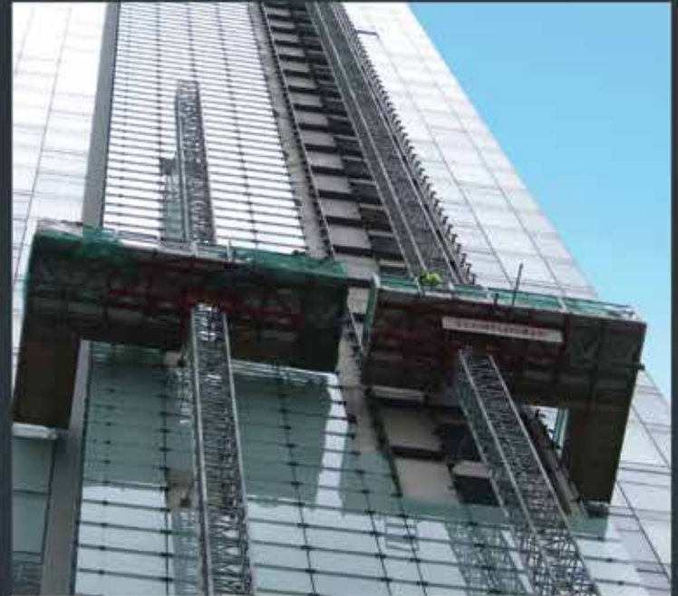
Heavy Duty Mast Climbers Tower West, Liverpool
