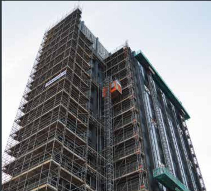
Double Stacked Mast Climbers Archway Tower
