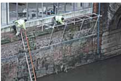
Working over a canal.
