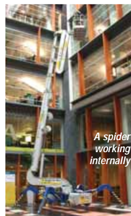
Sometimes the only way in is being lifted by a crane
