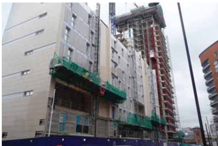
A Stross single mast passenger hoist on the Alberta House project
