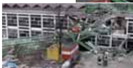
Strong winds all over Europe in mid January brought down this crane in Utrecht
