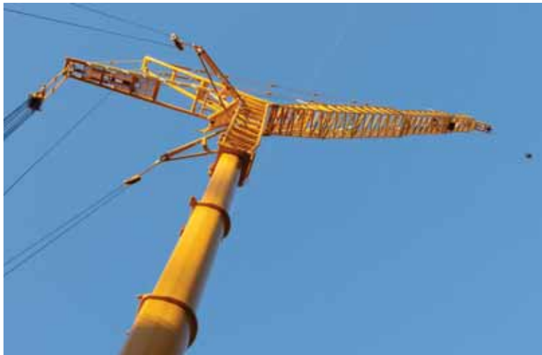
Fully rigged, the crane is huge
