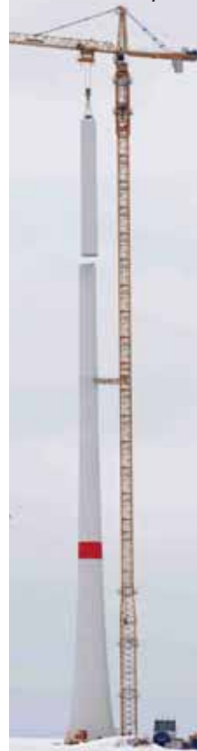
The top tower section is lifted into place
