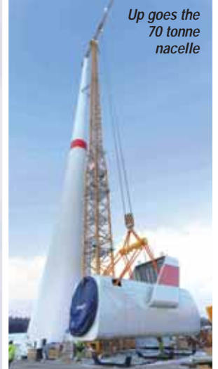
A mobile crane unloaded the parts and assembled the crane at its initial height of 50 metres
