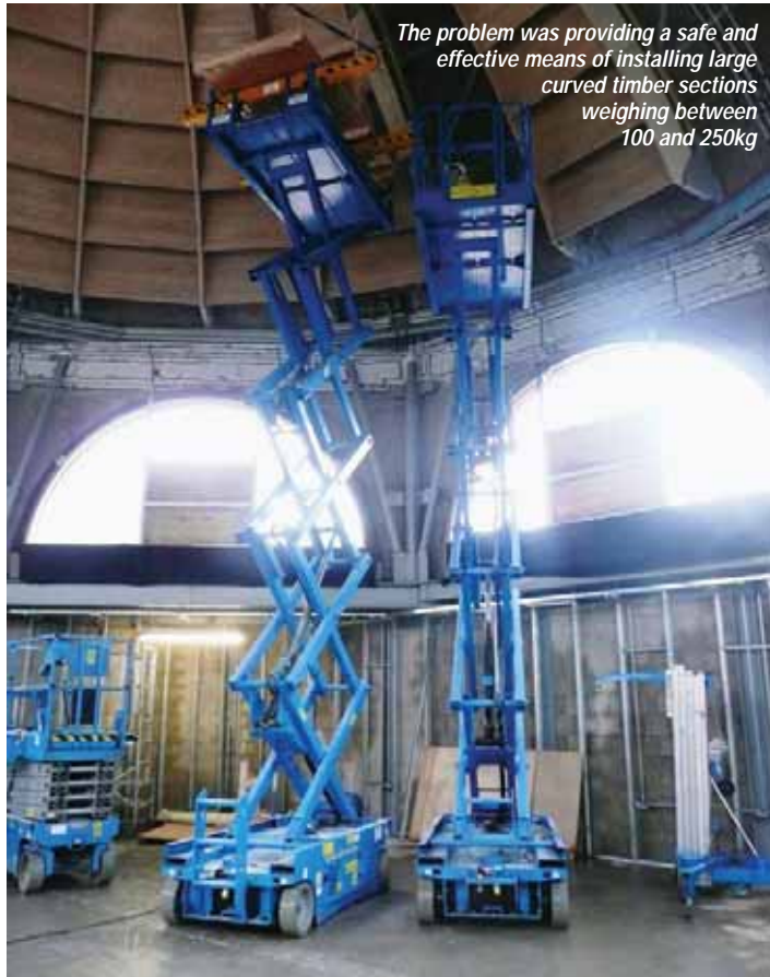
Nationwide Platforms supplied this SkyDuct attachment fitted to a modified Genie GS2646 scissor lift, capable of holding up to 350kg of materials without risk to operators or materials falling to the ground.
