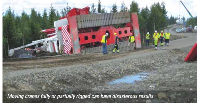
Many wind farm roads are too narrow and not designed to take rigged cranes
