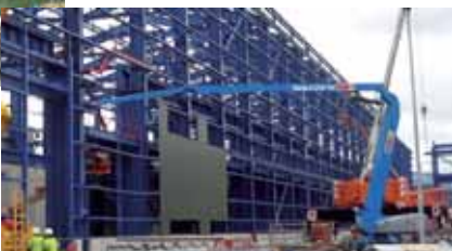
A Riwal 1250AJP at work at the Mosjøen plant, not exactly using its maximum work height
