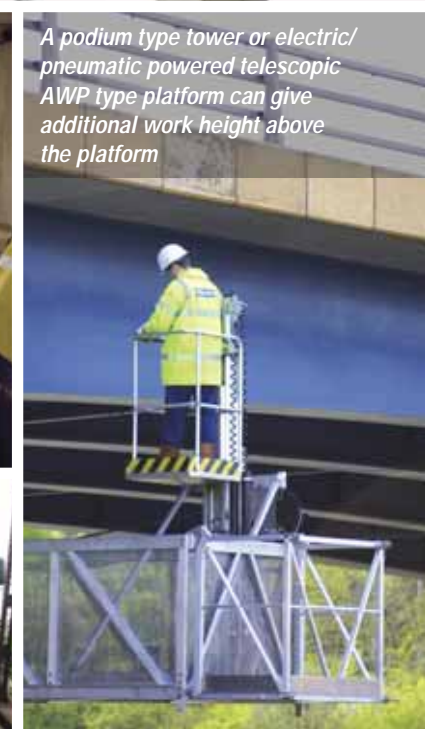
Platform for extending deck units provide a large work/inspection area
