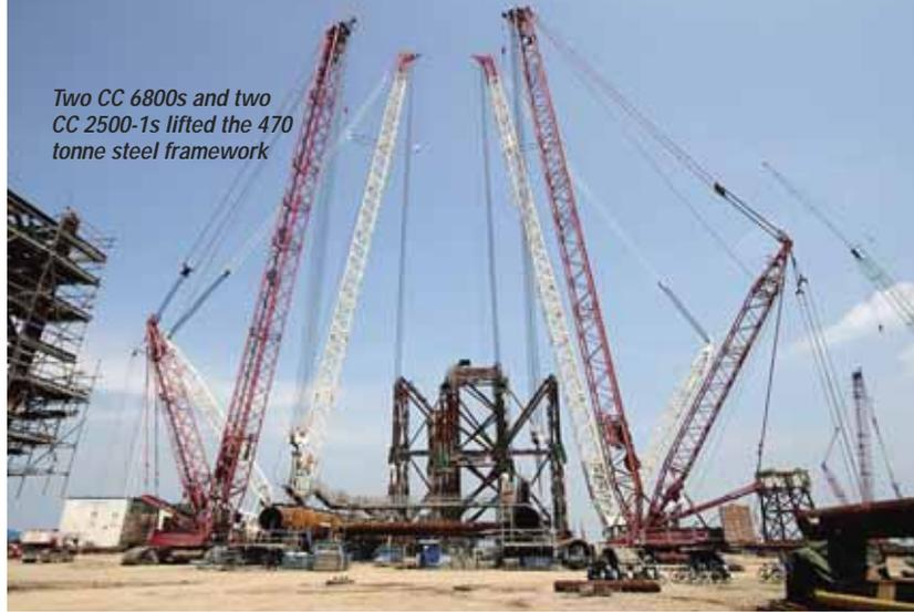
Two CC 6800s and two CC 2500-1s lifted the 470 tonne steel framework
