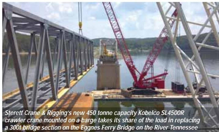
Sterett Crane & Rigging's new 450 tonne capacity Kobelco SL4500R crawler crane mounted on a barge takes its share of the load in replacing a 300t bridge section on the Eggness Ferry Bridge on the River Tennessee
