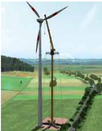
The GTK1100 telescopic tower crane is delivered on four trucks
