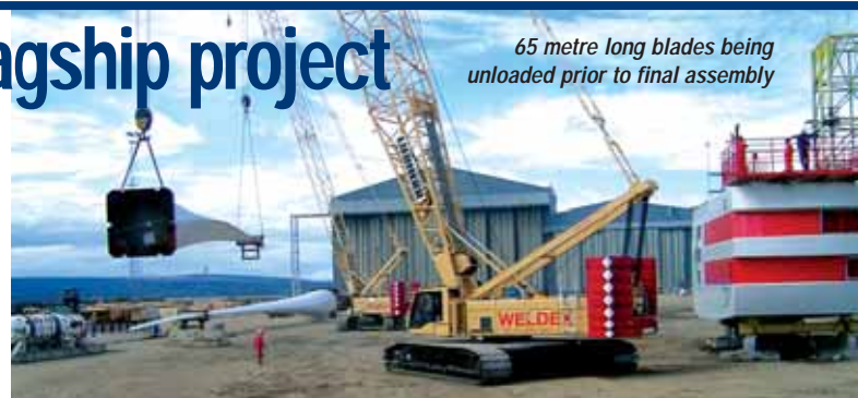
When travelling the side outriggers can be lifted giving a 5m track width
