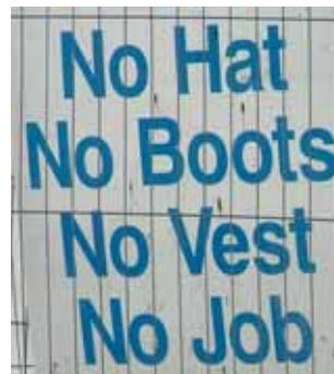
Boots, hats and yellow vests but no harnesses in boom lifts
