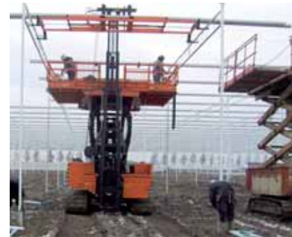
On this special, the building frames are loaded on the material lift... and lifted into place for fixing.
