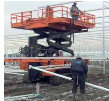
On this special, the building frames are loaded on the material lift... and lifted into place for fixing.
