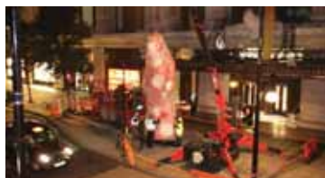
The 6m high statue installed
