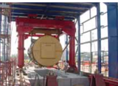
ALE's jacking system installs one of the gas turbines over the generator foundation at the power station in Turbigo, Italy
