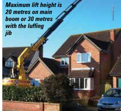
**Maximum lift height is 20 metres on main boom or 30 metres with the luffing jib**
